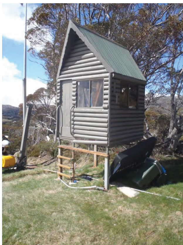
Figure 6: Existing hut to be removed
